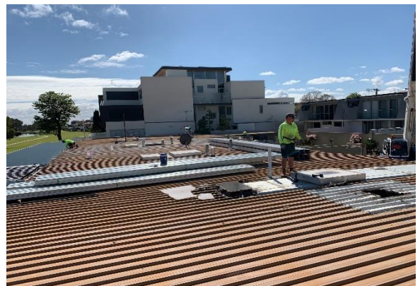
Image 2: Roof works midway
