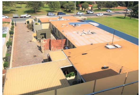
Image 1: Overhead view prior to works
