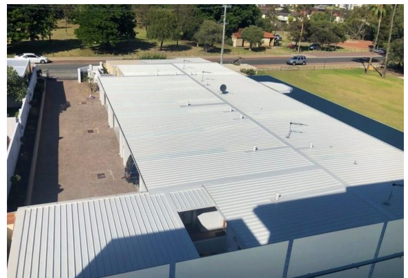
Image 3: Works at completion
