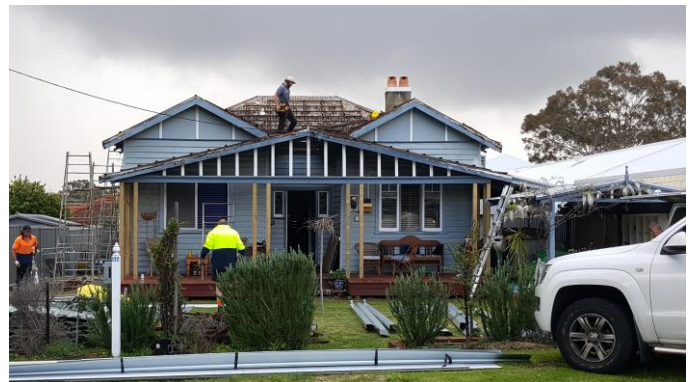
Image 2: Mid repairs and new roof installation
