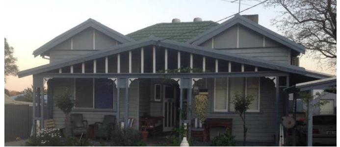
Image 1: Street view prior to work commencement
