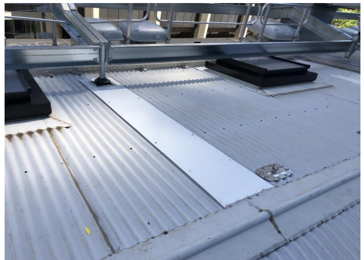
Image 3: Dry pan flashings will provide long-term water tightness
